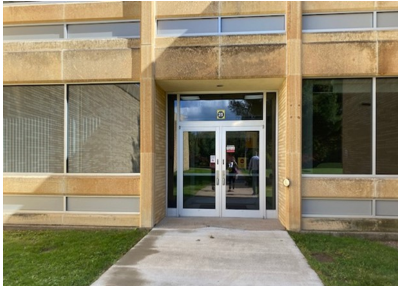
Dedicated UW-Eau Claire entrance to the Helen Connor Laird Fine Arts Building on the UW-Stevens Point at Marshfield campus, signage pending
